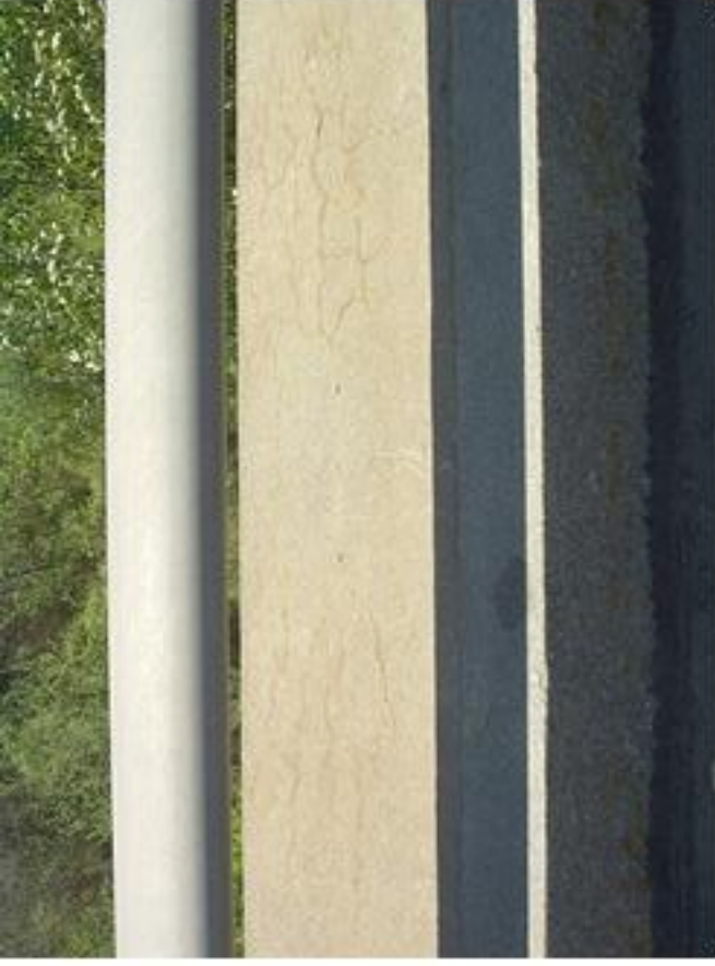
Cracking in curb typical.
