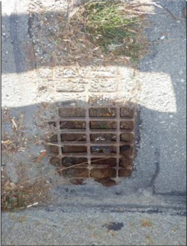
Partially plugged drains with rusted thru downspouts - Typical
