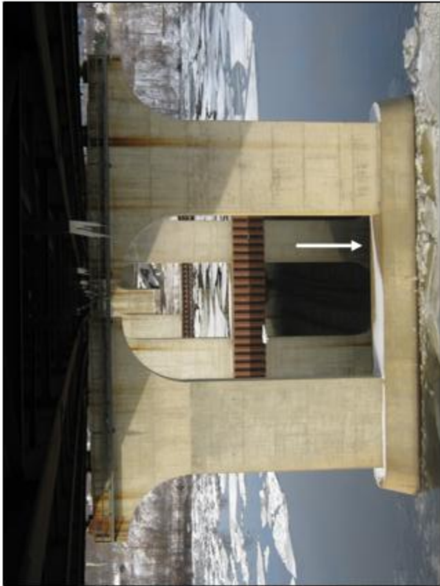
Pier #5 with visible large through crack at northern edge of footing
