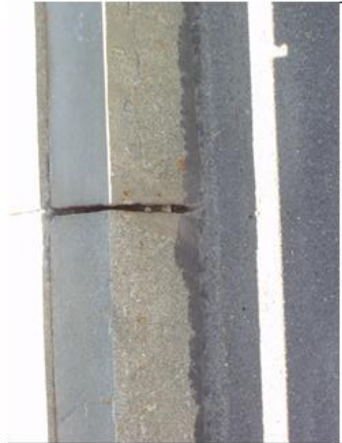
Pointing largely failed.
