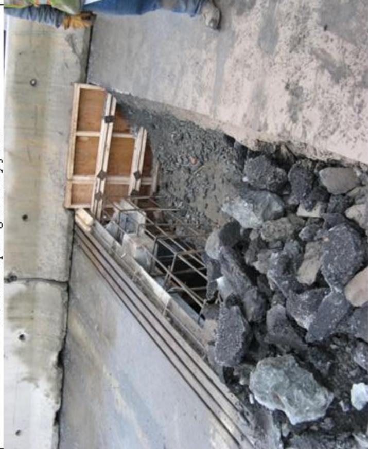
Br Maint rehab'g and retrofitting SE'ly joint.
