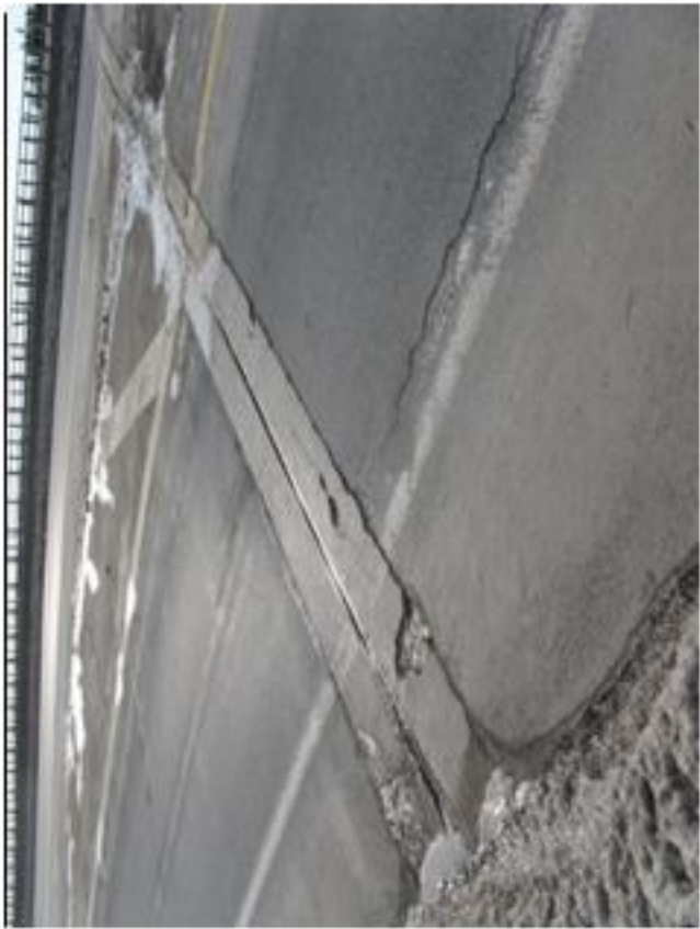
Potholes in westbound west joint header
