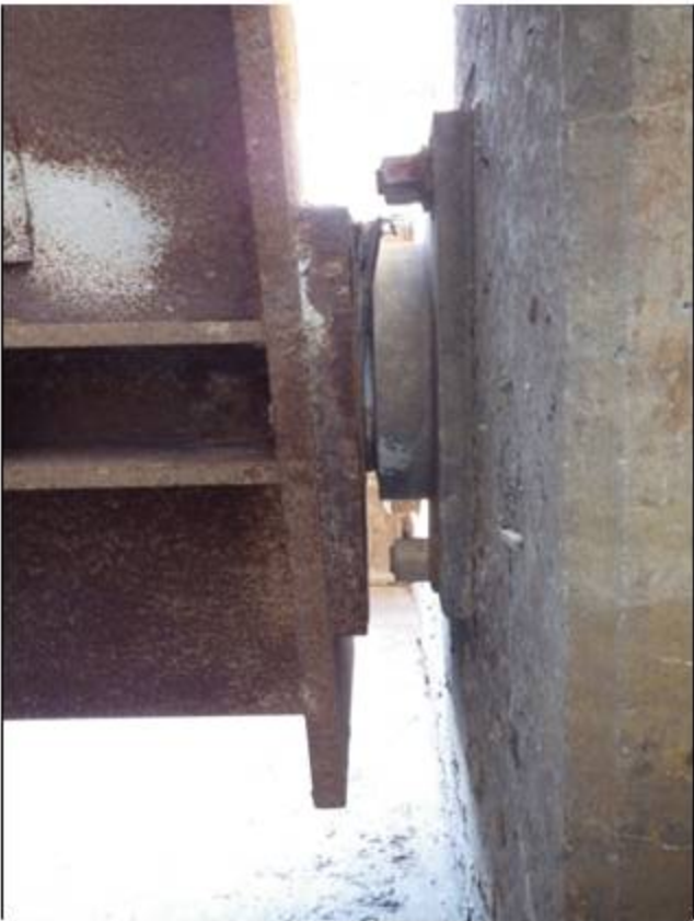
Bearings slid back approx. 6" with damaged slide plates
