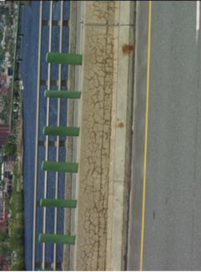
Typical cracking in barrier rail.
