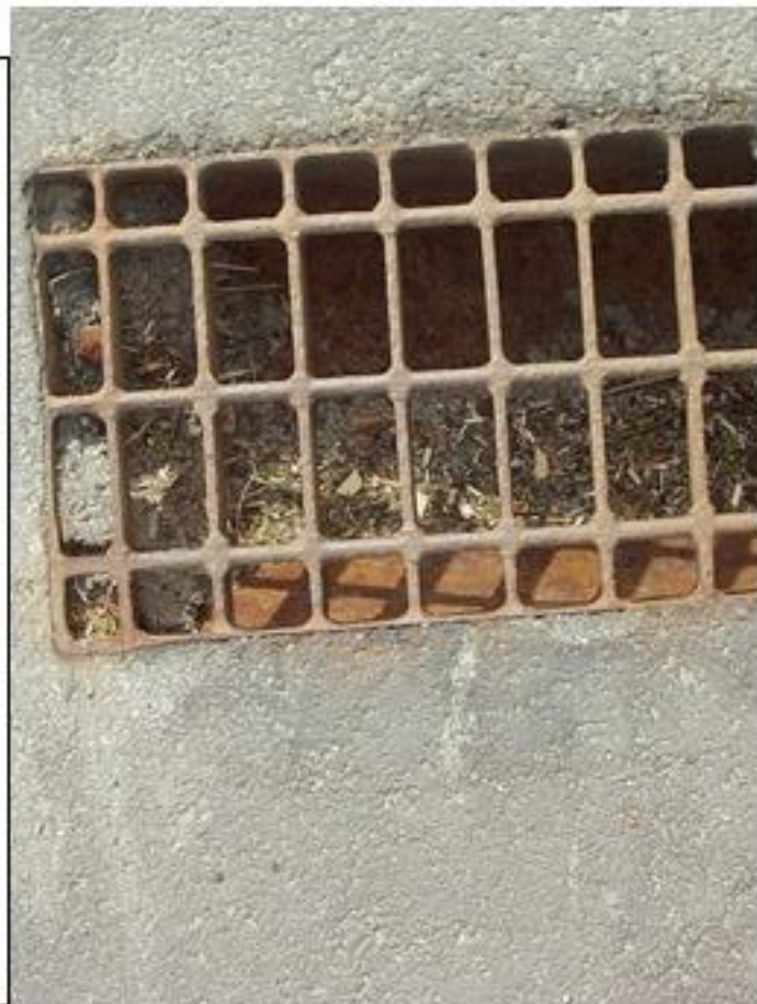
≤ or = severe sect loss at drain inlet.
