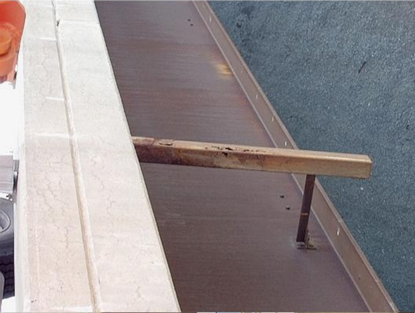
Multiple perforations in drain.
