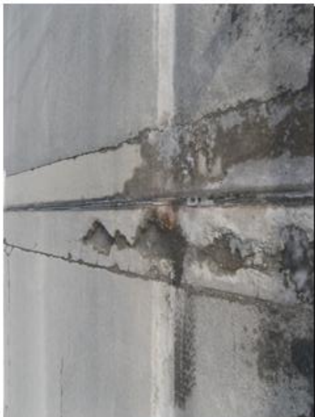
Small potholes in joint header
