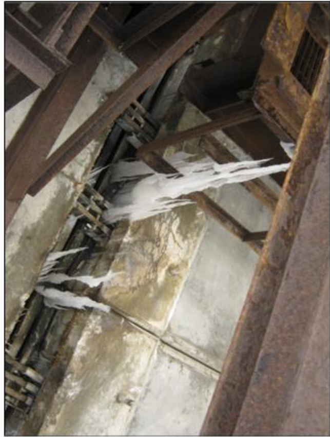
Failed seal with heavy corrosion of weathering steel and det. of concrete
