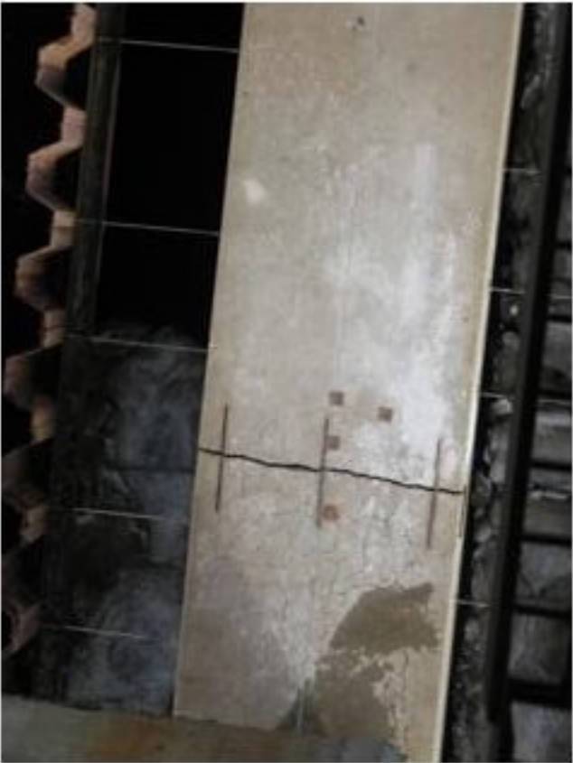
Documented crack in west channel pier footing
