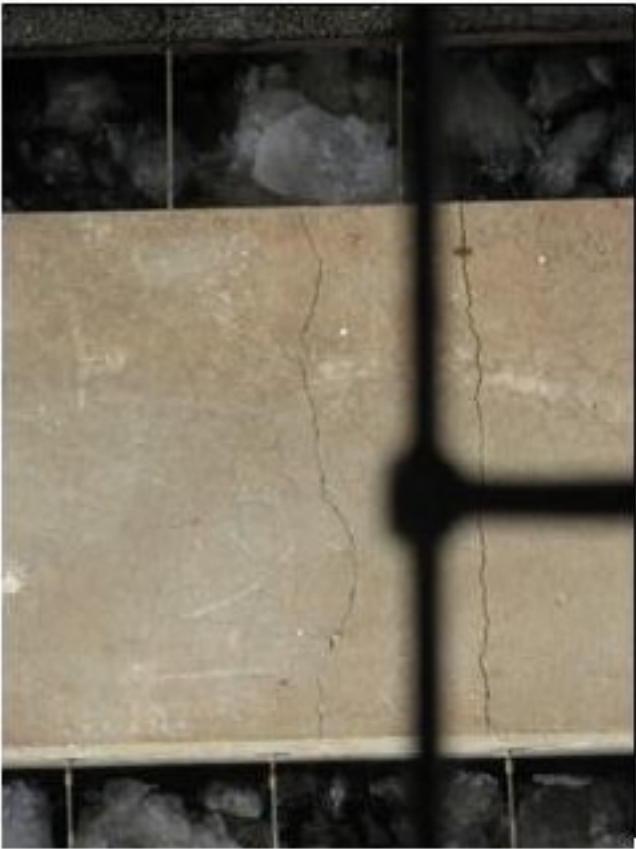
Crack in 2 nd westerly channel pier footing
