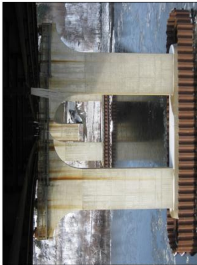
Typical river pier, note weathering steel rust washing down columns
