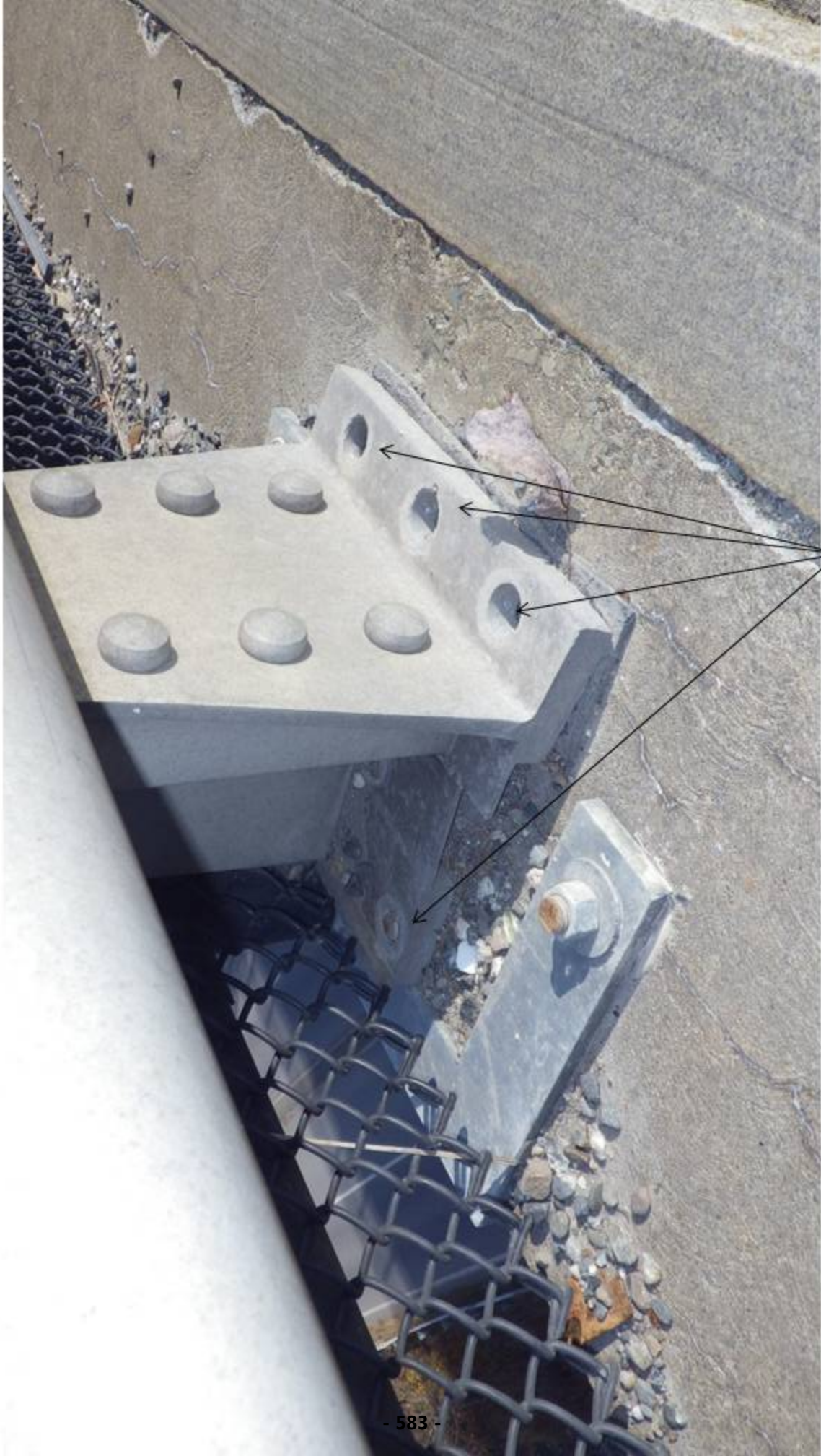
One post on the north side has four anchor bolts sheared off, leaving only one on the back side
