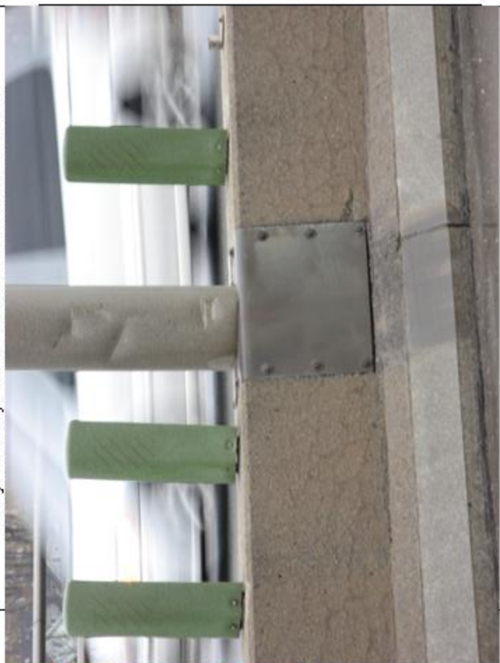
Light mast dam'd. Typ barrier cracking.
