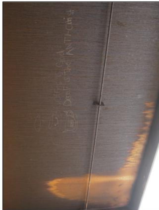
Abnormal weathering of steel at scattered locations
