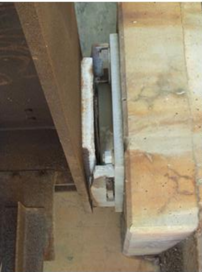
Bearing sliding surface delam'd...
