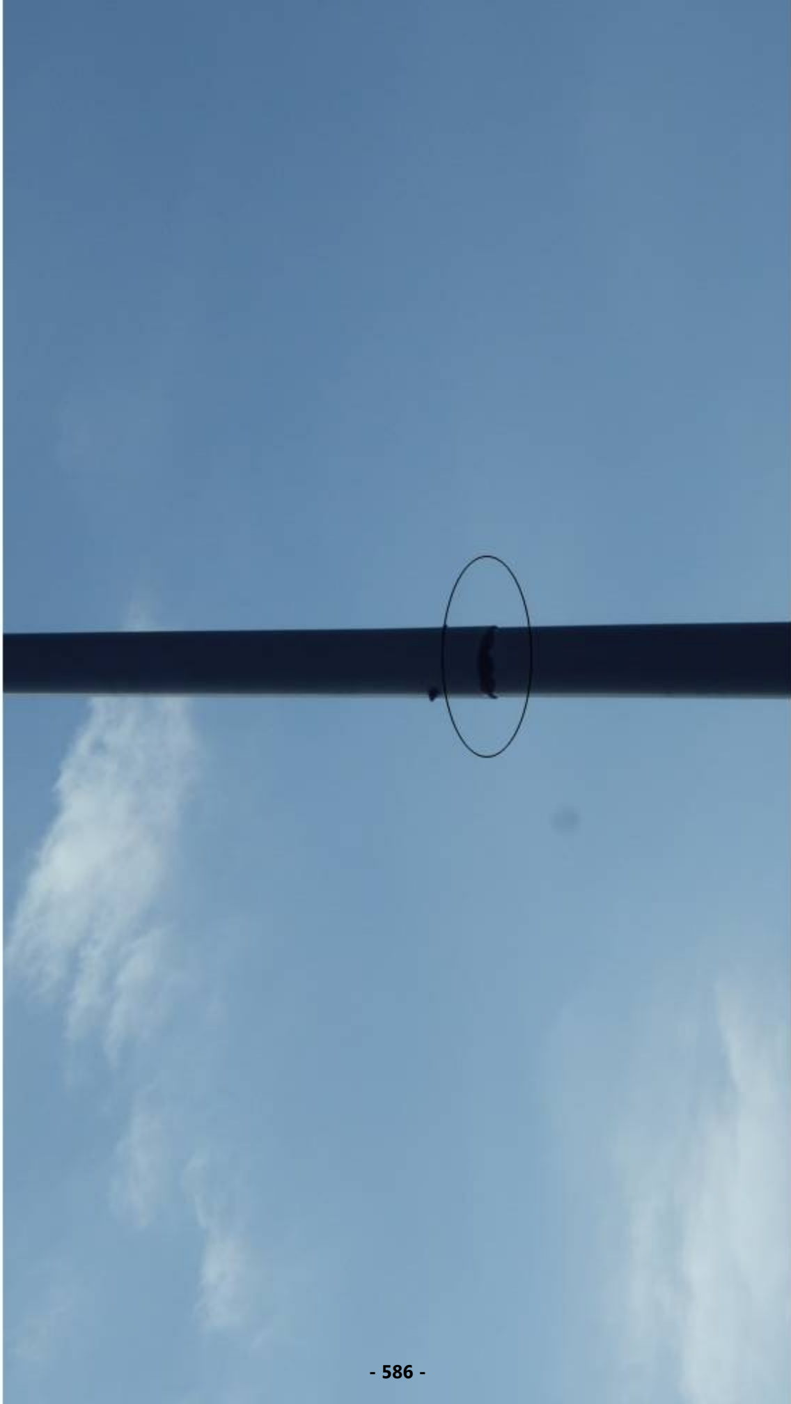
First median light post from Brewer side has t slip joint
