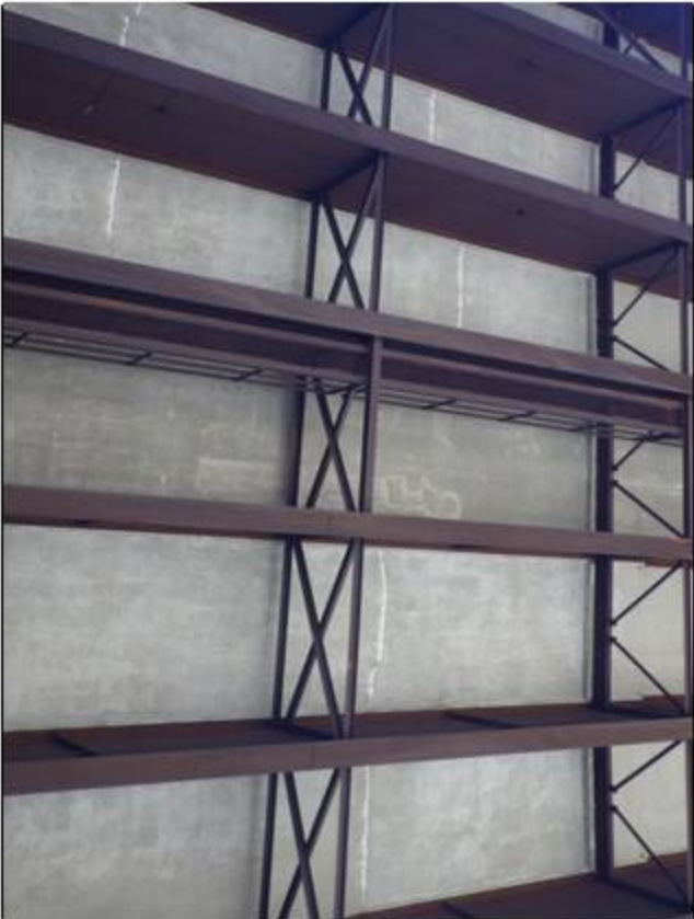
East span - Scattered minor transverse cracking with light efflorescences
