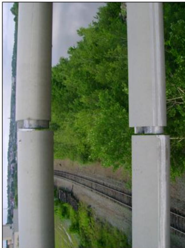
Bridge rail splice disconnected (approx. over Pier #2 westbound)
