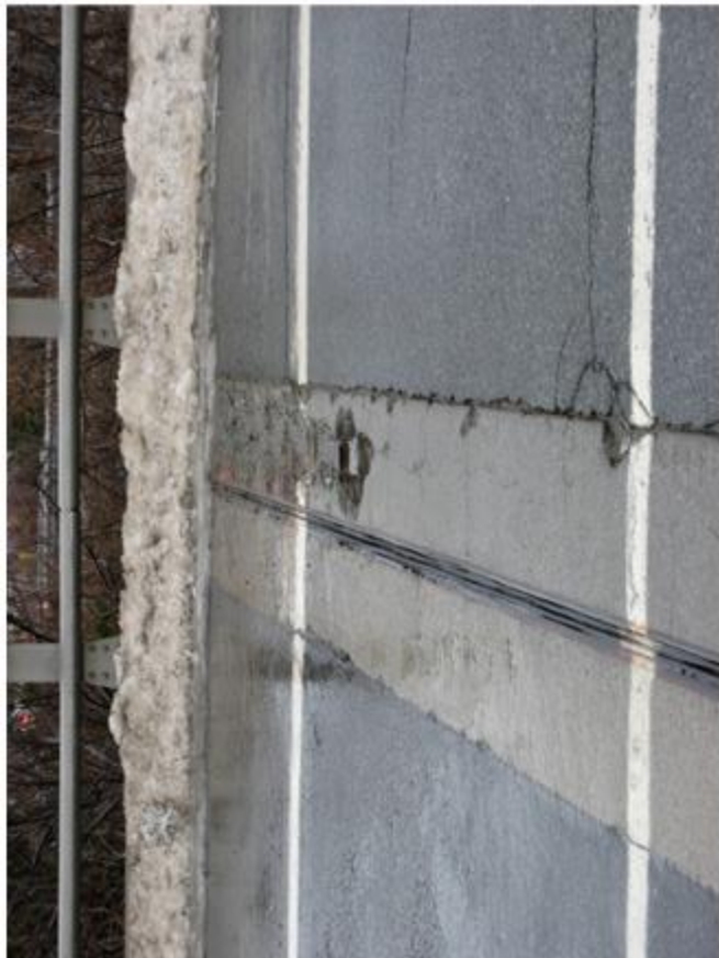
Isol'd sev spalling of NW'ly joint.
