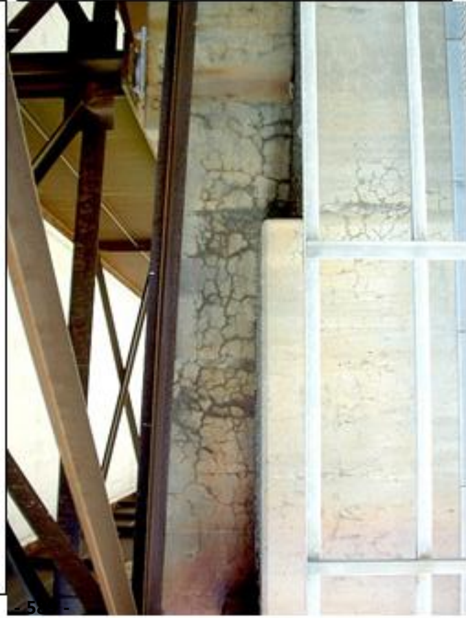
Deterioration of pier below leaky deck joint.
