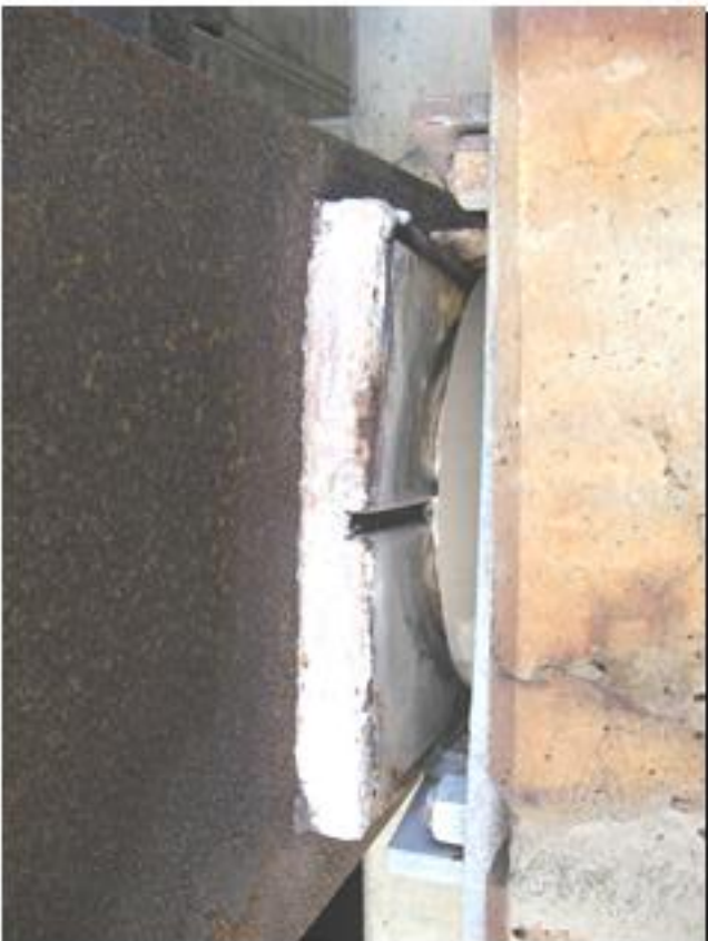
Corroding at bearing top plate west pier
