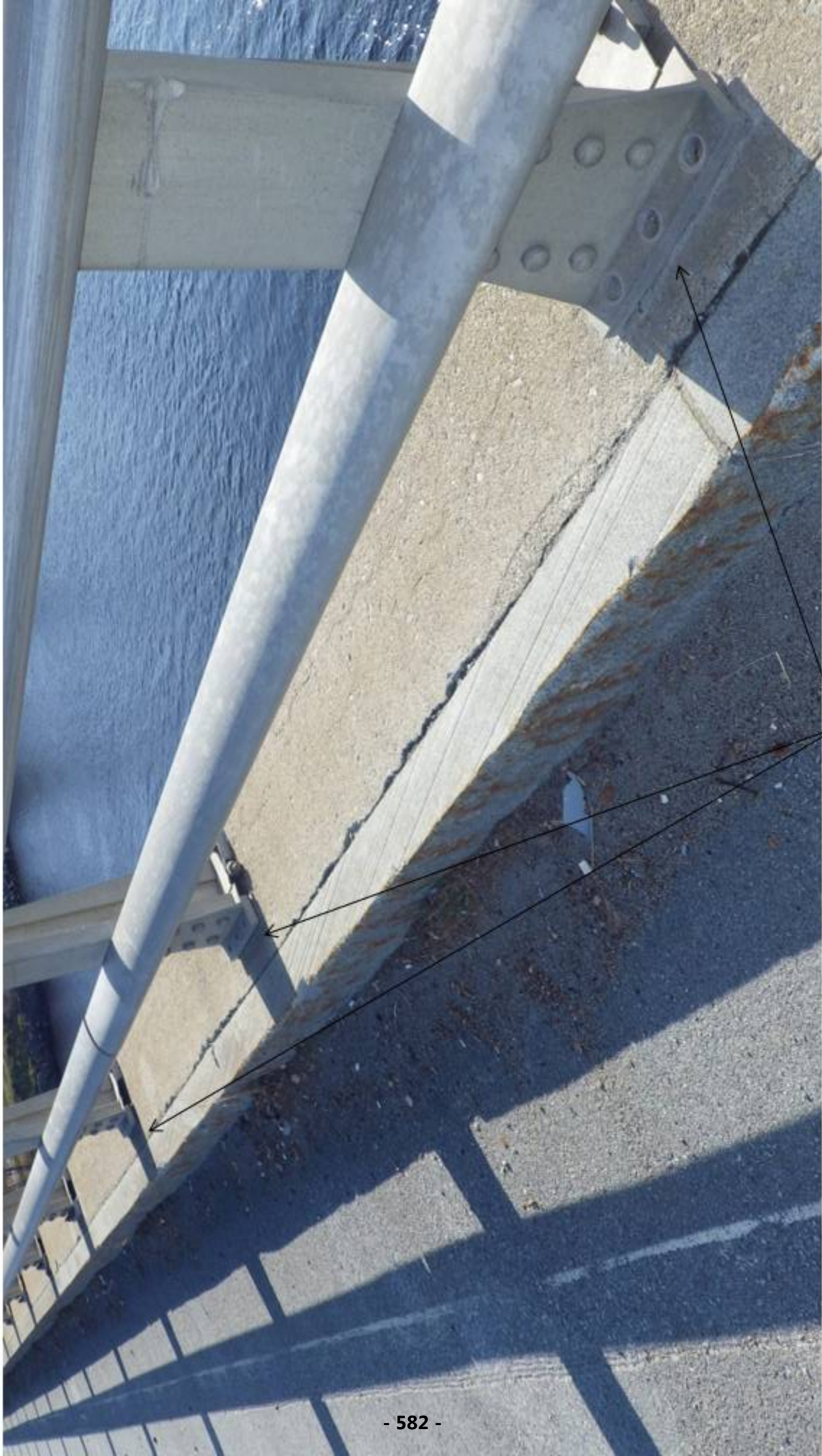
Bridge rail post with the three front anchor bolts sheared off and only two on the back – Eleven on the south side and five on the north side – Some of these areas span two to three posts, diminishing the strength of the rail if impacted
