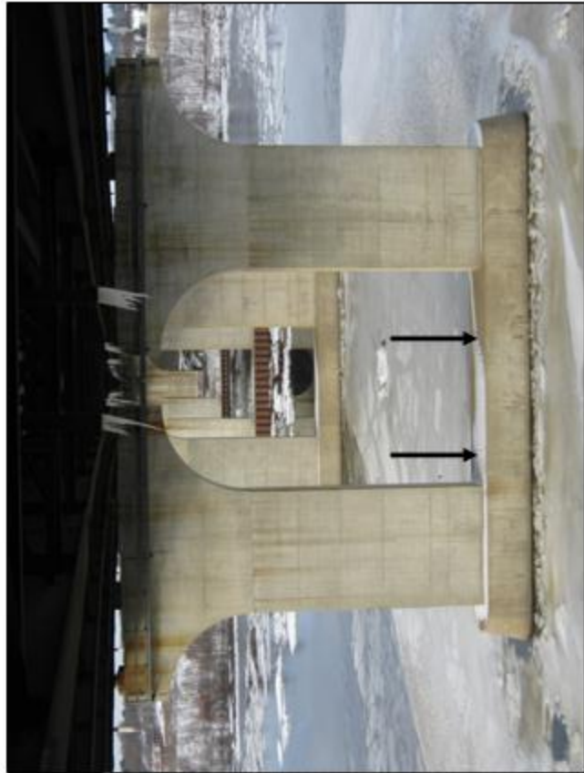
Easternmost water pier (#6) with multiple large footing cracks
