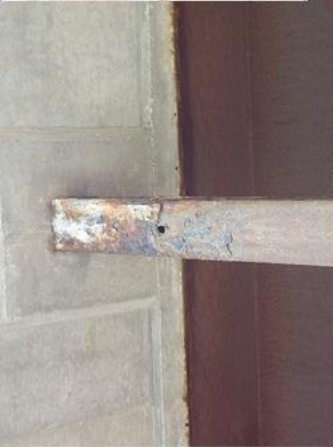
Perforation in drain.
