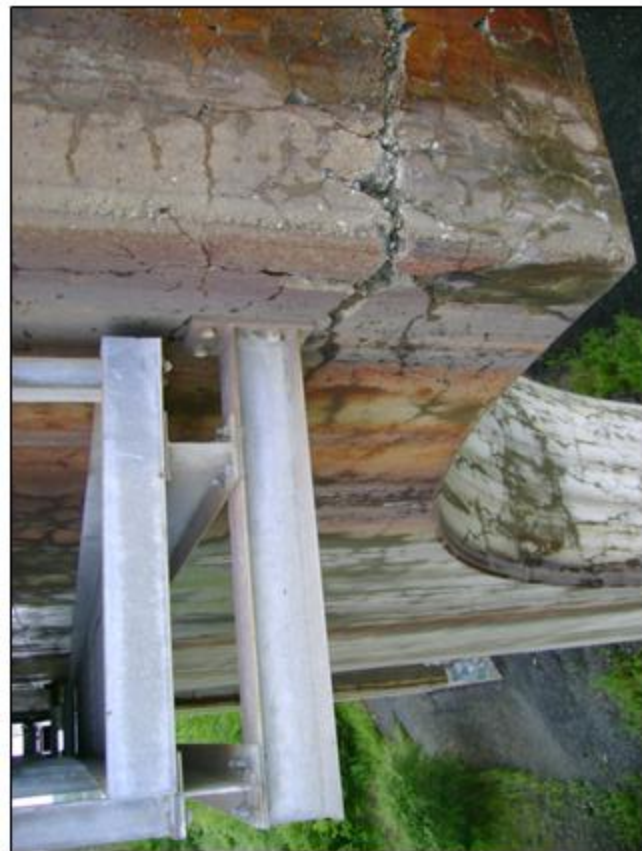
Deterioration of concrete at Pier #2, northeastern corner
