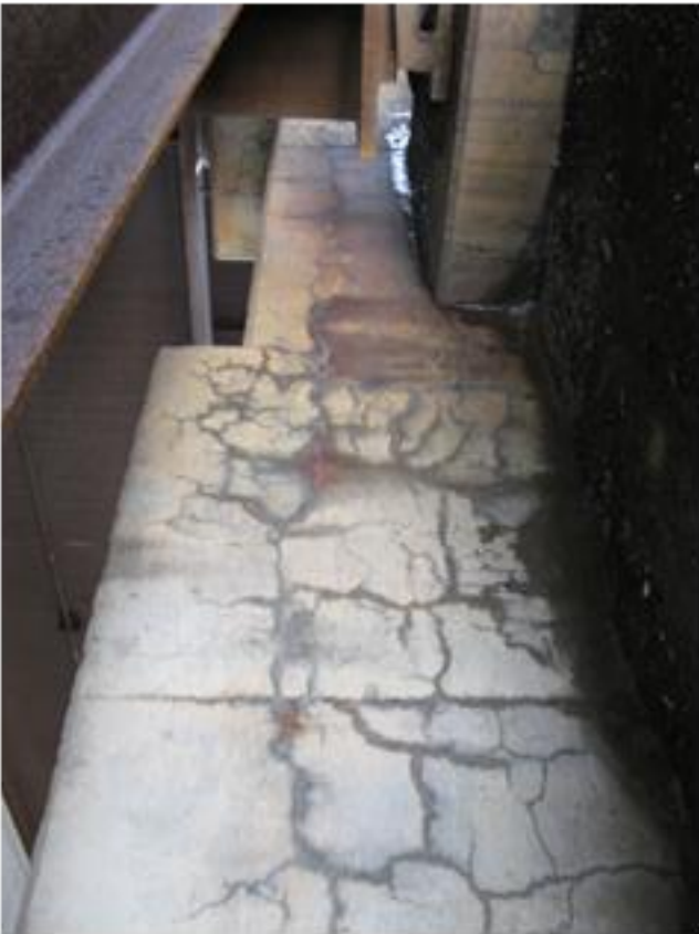
Cracking concrete with rust staining Abutment
