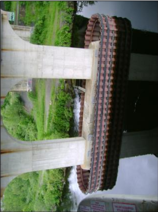
Westernmost water pier (#3) with footing post tension strengthening
