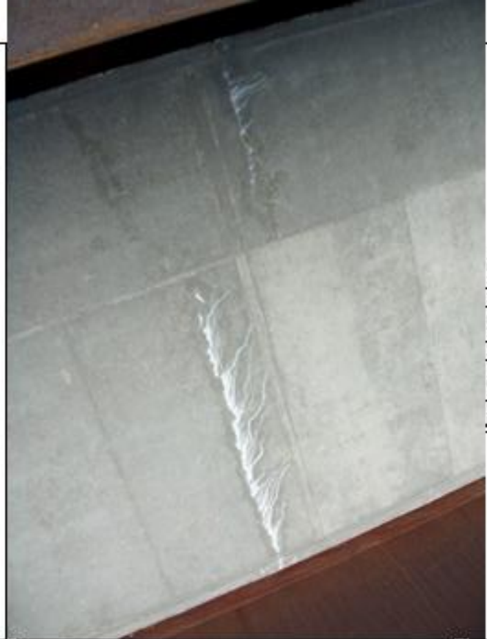
Pointing largely failed.
