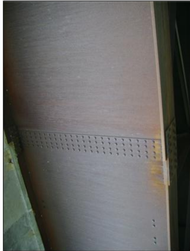
Typical beam splice
