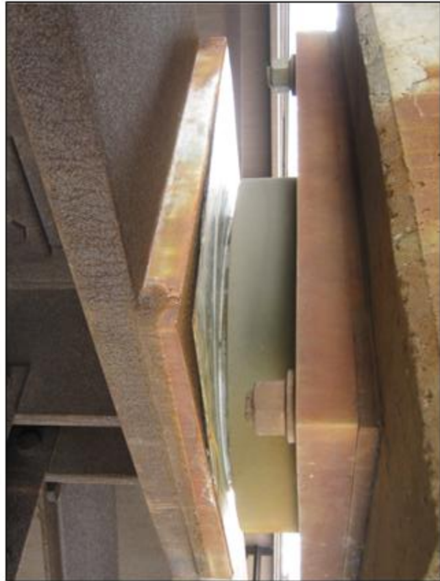
Typical bearing with some delamination of friction plate
