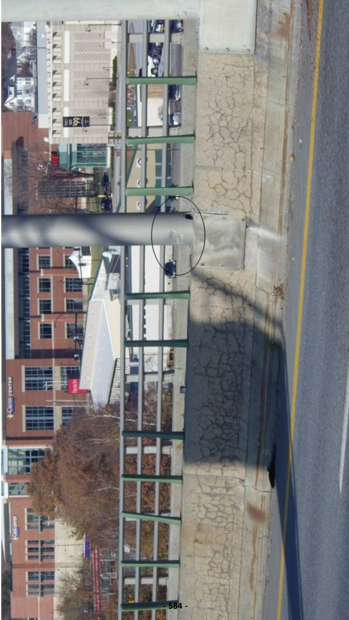
First median light post from Bangor side has impact damage
