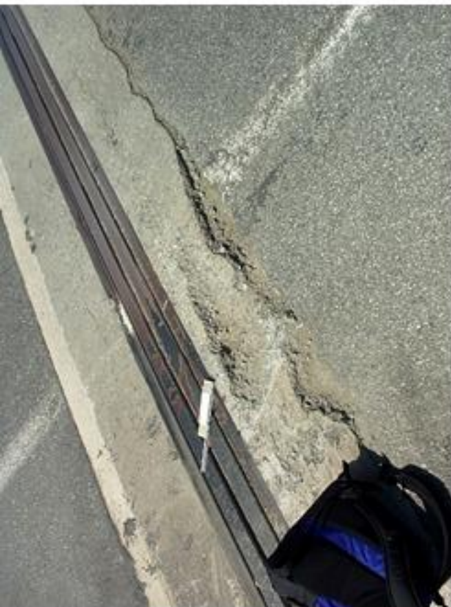
Section loss in joint bulkhead to 2 5/8 in penetration.
