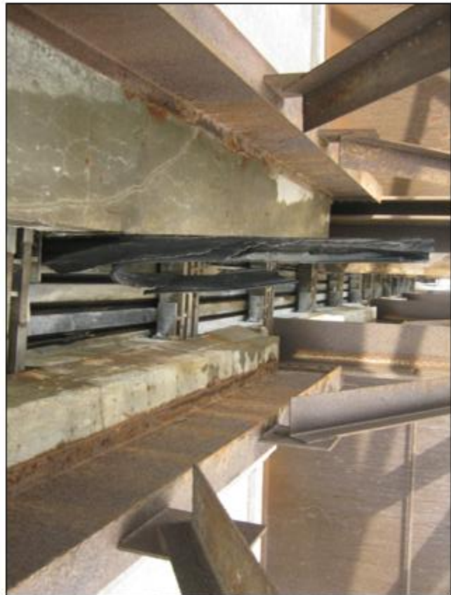
Failed bridge joint seal over Pier 2
