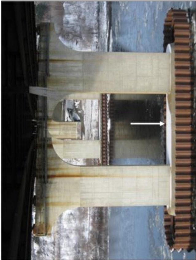
Pier #4 with large crack through crack at center of footing
