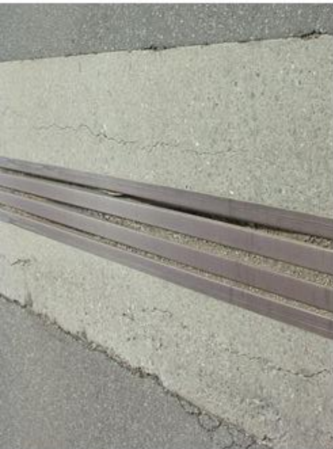
Typ cracking in E'ly modular joint.
