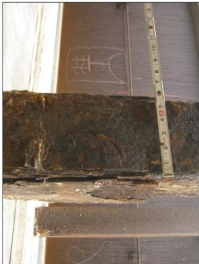
Corrosion of bridge drains - typical of approximately half
