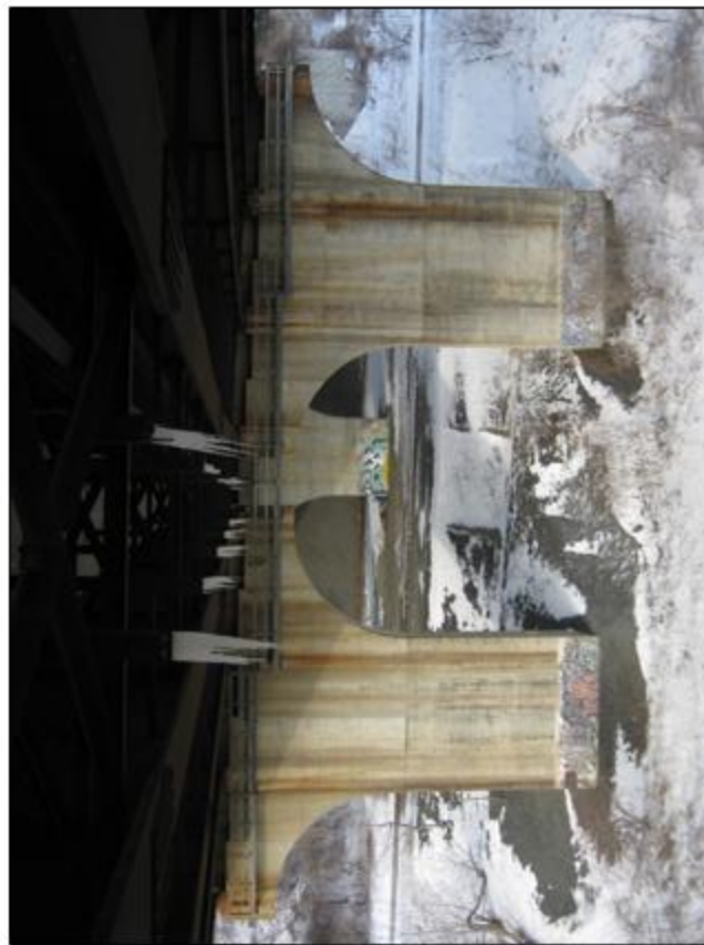
Typical land pier, note weathering steel rust washing down columns
