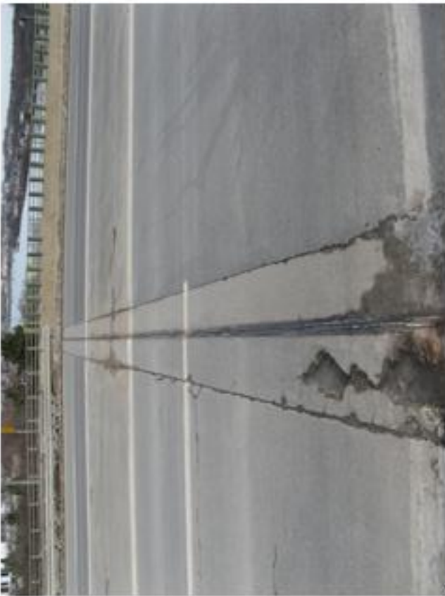
Small potholes in joint header
