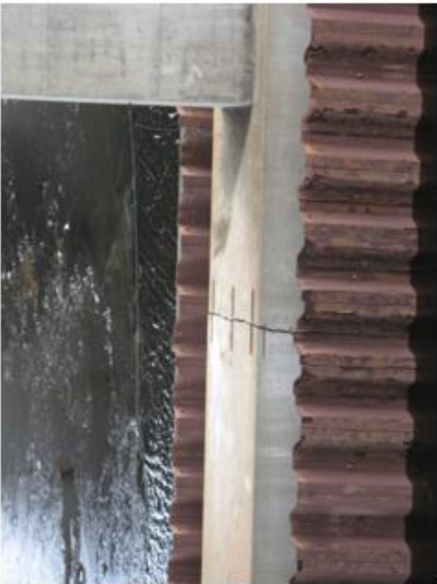
Documented crack in west channel pier footing
