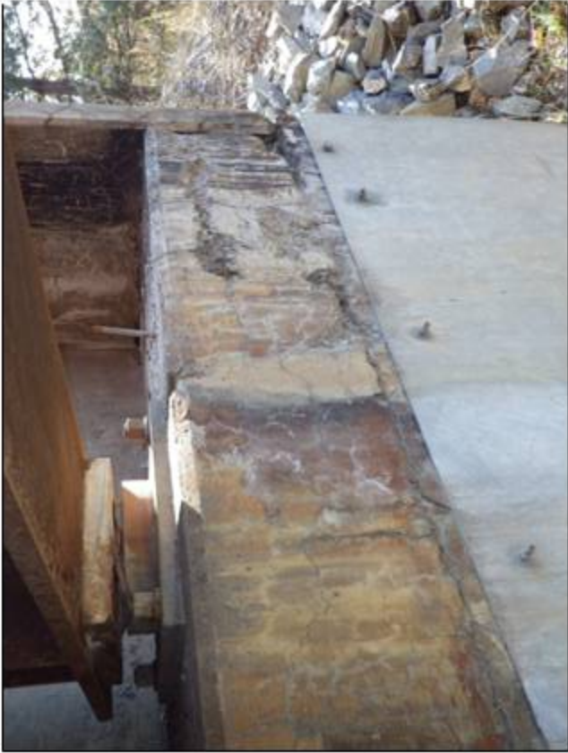
Bearings slid back approx. 6" with damaged slide plates
