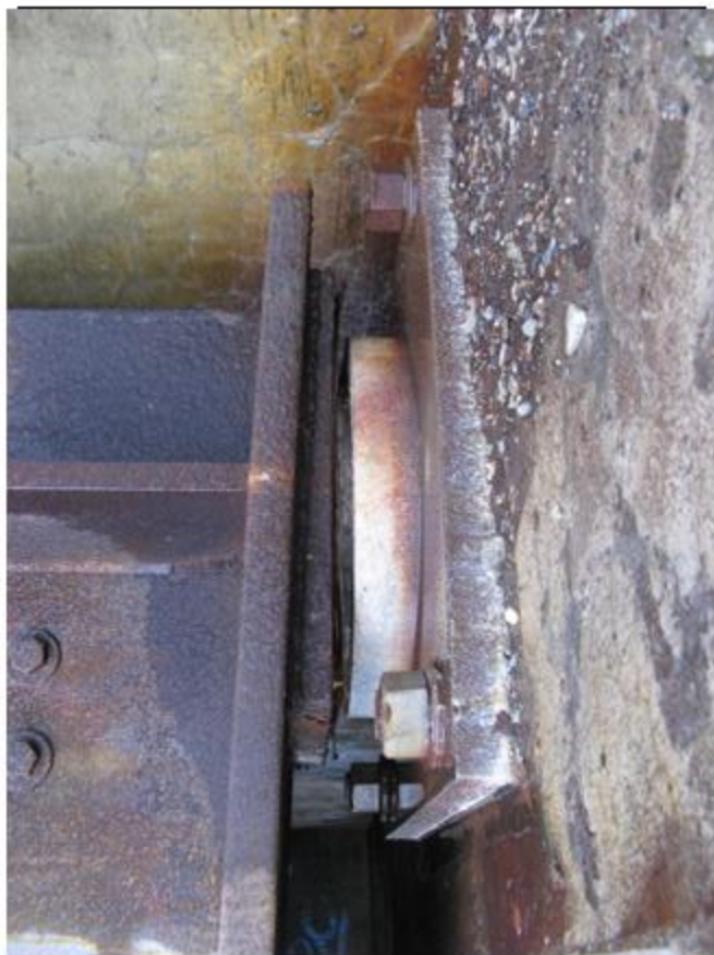
Sliding surface broken free from sole plate – freq problem of some area.
