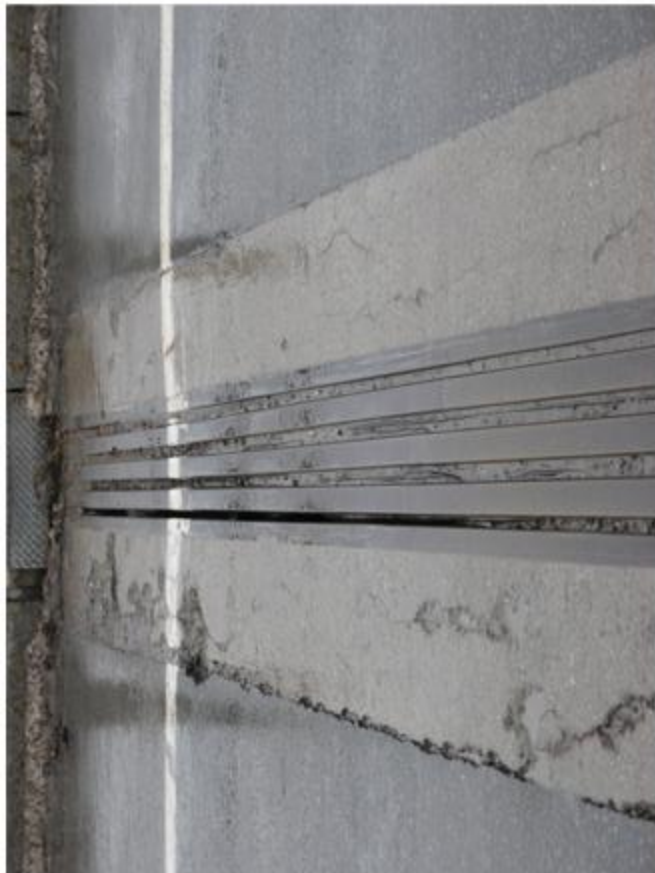
NW'ly modular joint: dam'd bulkhead + one of seals failed.
